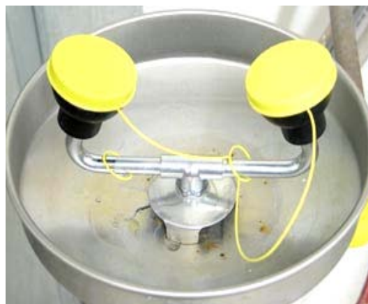
Fig. Emergency Eyewash Unit
